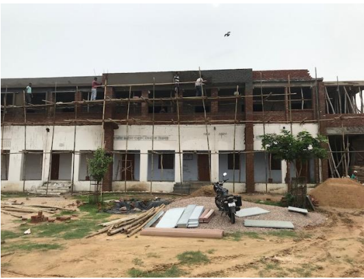
Sardar School, Jaipur – work almost completed
