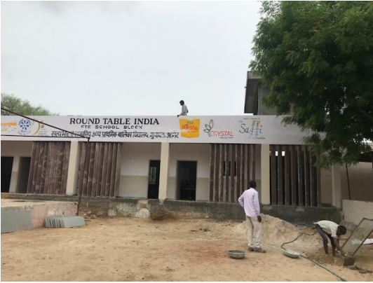
Satya Bharti School, Jaipur – work almost completed
