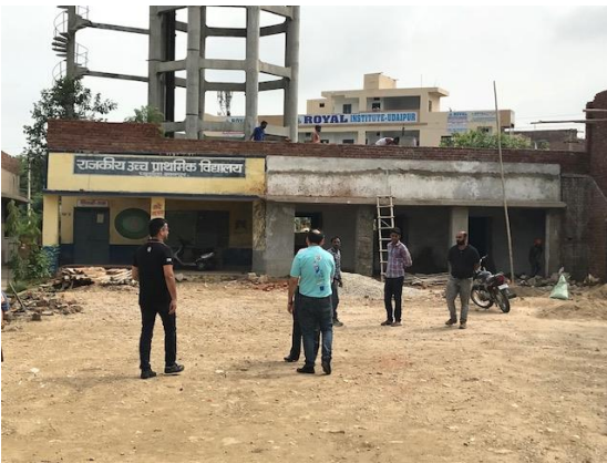
Pahada School, Udaipur – work almost completed
